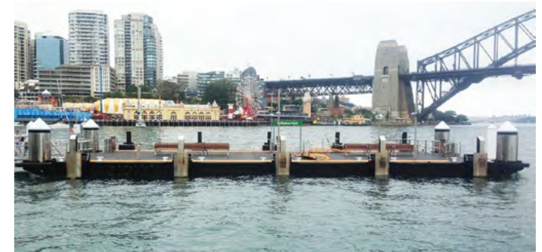
MCMAHONS POINT FERRY WHARF, SYDNEY The piled floating pontoon
