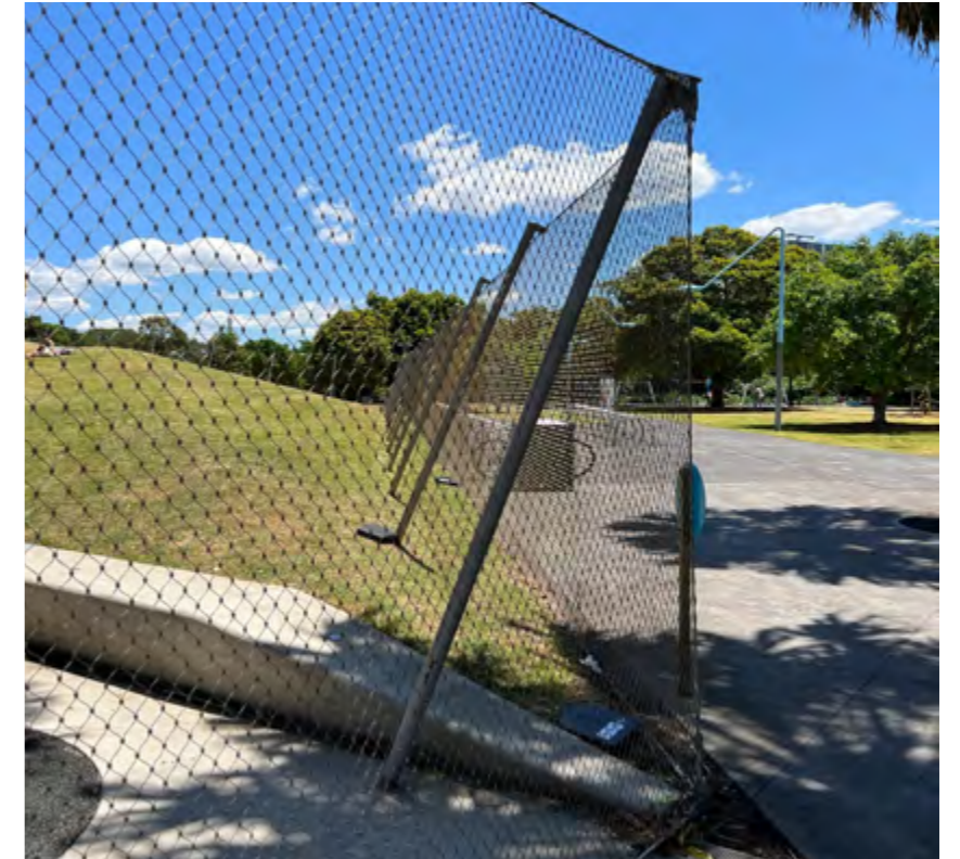
PRINCE ALFRED PARK POOL, AUSTRALIA Secure but unobtrusive steel perimeter fencing allowing a seamless connection with the landscape Image - Studio Octopi
