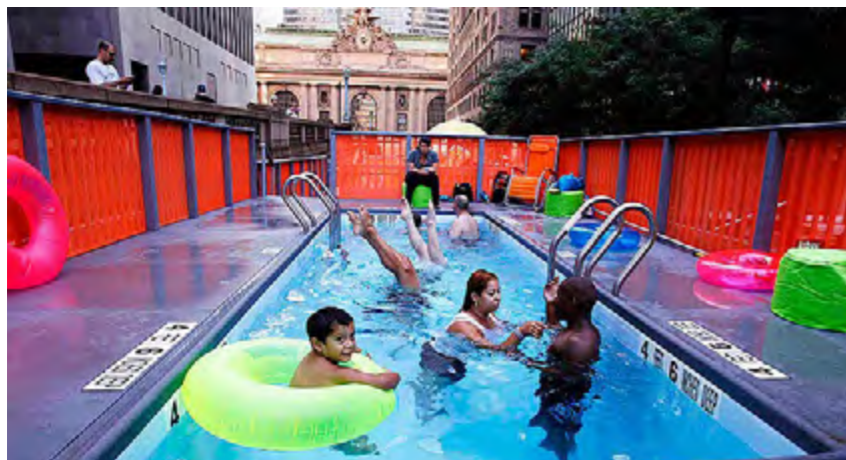
DUMPSTER POOLS, USA Only 10 people could swim comfortably at a time. Each 8 x 22 ft dumpster pool was surrounded by a wrap-around deck and had its own built-in water filtration system
