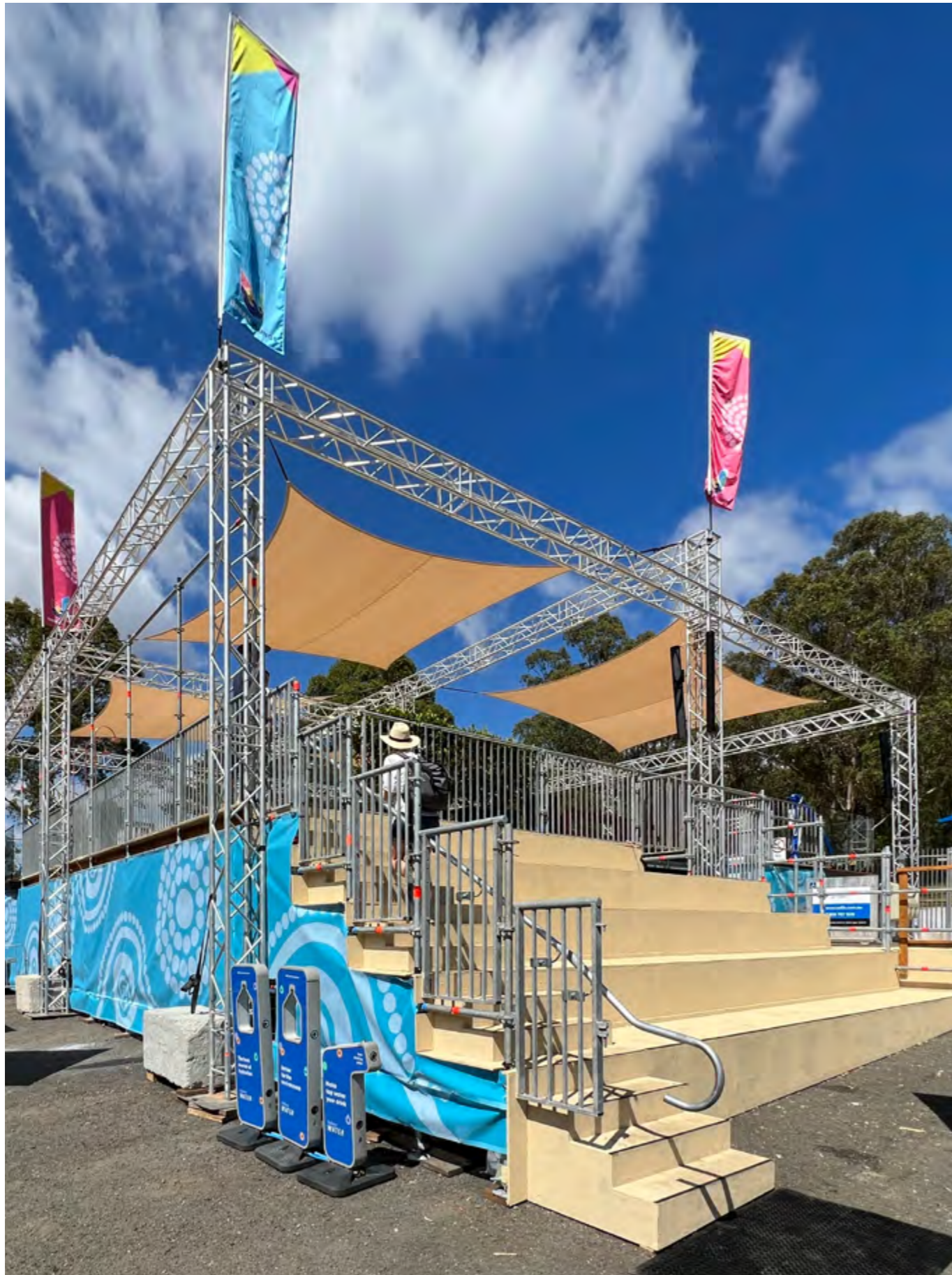
CONCEPT 4 Designed to use off the shelf shade cloths and scaffolding to reduce cost and reduce construction time
