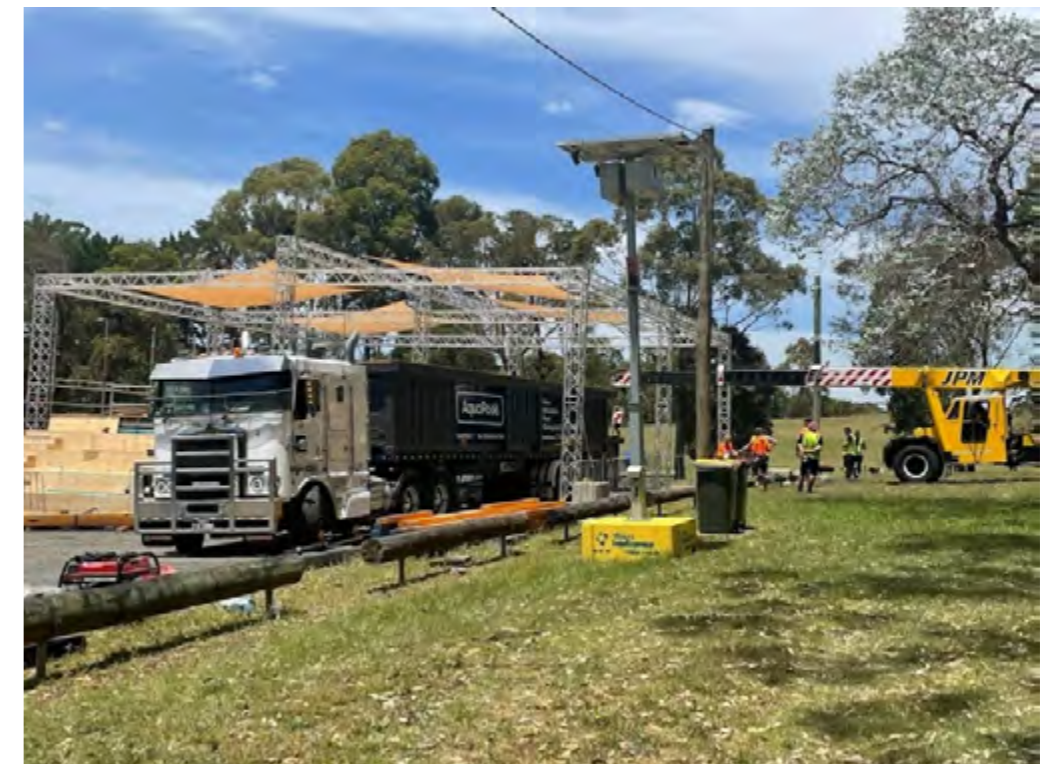
CONCEPT 4 Second container pool craned into position
